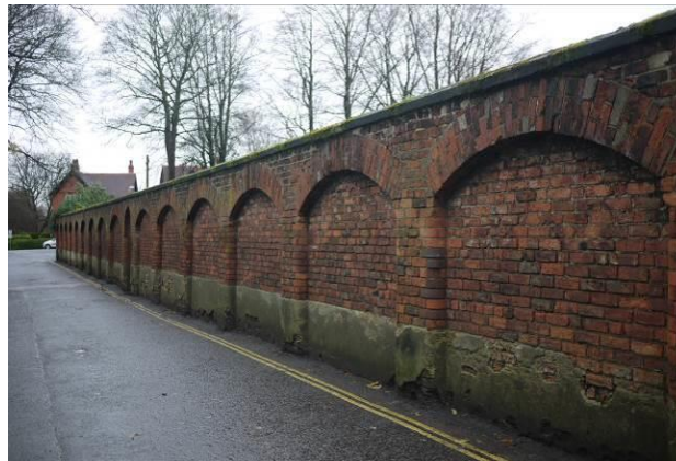
Rear wall of the walled garden area
