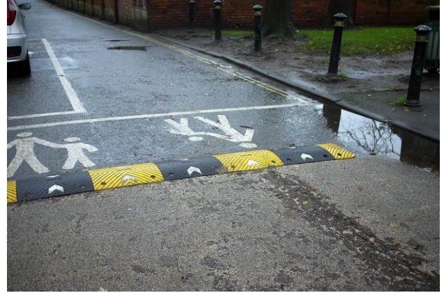
Intrusive speed bumps
