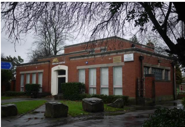
Former Firwood Library on Kings Road
